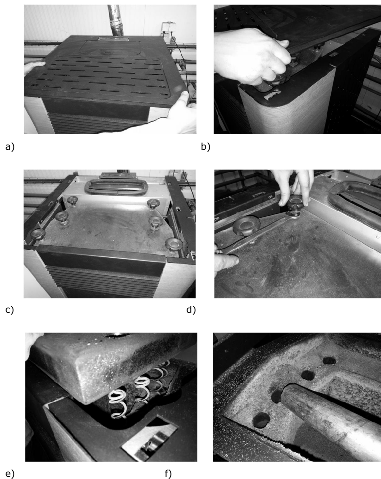
Figure 35 – Cleaning of gas passageways and turbulators
