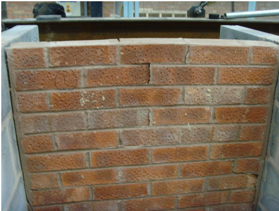
Plate 1 Flexural Failure of Wall One
